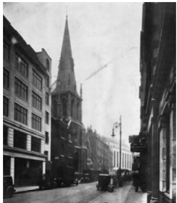
Fig. 4 St. Andrew's Church, Wells Street, London, by S. W. Daukes and Hamilton. 1847. National Monuments Record, Swindon .
